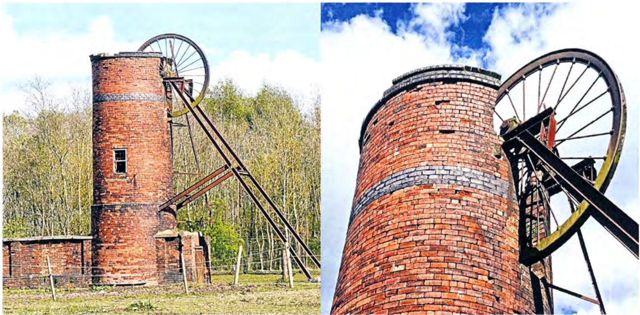
Plates 18 & 19 Brittain Pit, Swanwick dating from the 19 th century now forms part of the Midland Railway Centre near Butterley. This would probably have been the upcast shaft.
