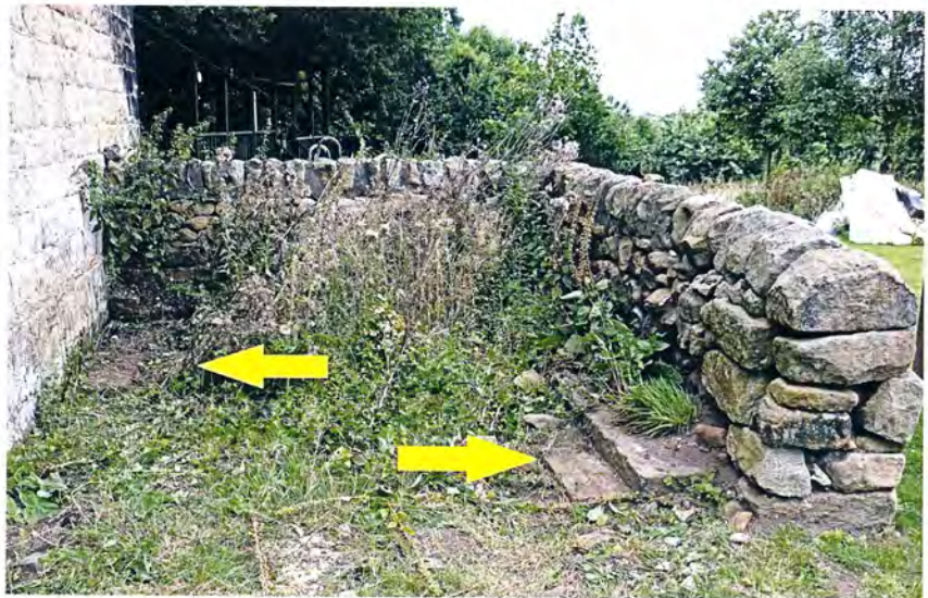
Plate 6 The enclosed space adjacent to the east wall. The arrows indicate the two lines of brickwork.
