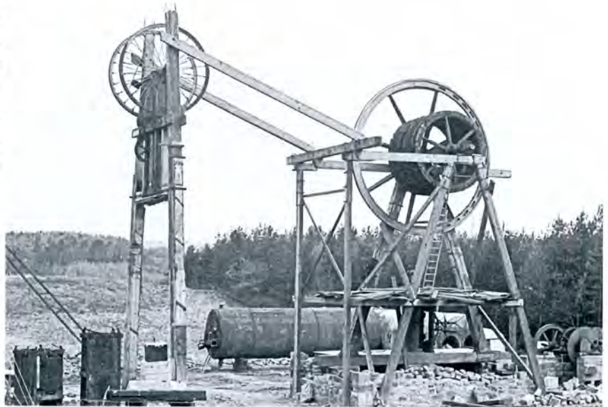
Plate 16 The ex Chophill Colliery engine of 1855 under re-erection at Beamish c1974. ( http://beamishtransportonline.co.uk/2015/01/remembering-frank-atkinson )
