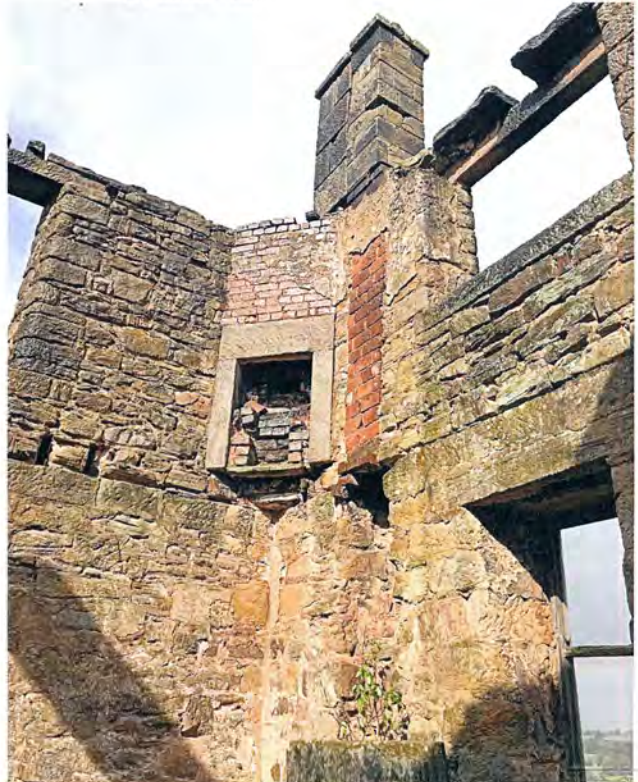
Plate 23 This fireplace is possibly evidence of alterations from its period of domestic habitation.
