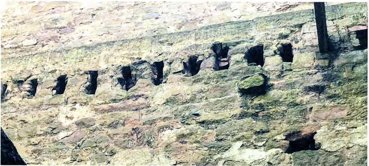
Plate 14 Holes inserted for later flooring arrangements.
