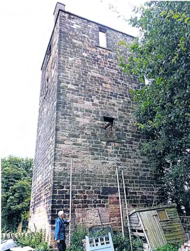
Plate 21 The north wall of the tower.
